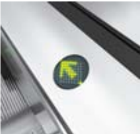
Traffic lights located in the decking
