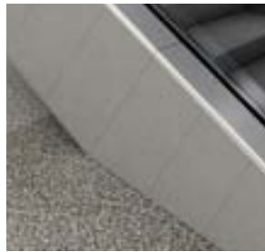
Grey powder coated sheet steel cladding (RAL7036)*****
