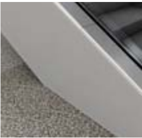
Grey primed sheet steel cladding (RAL7036) *
